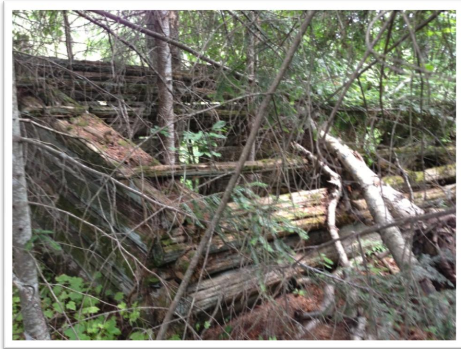
Figure 4. Second structure with trees encroaching on exterior and interior.
