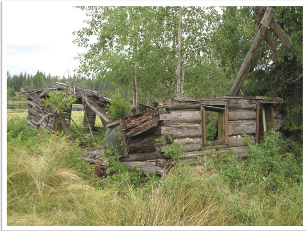
Figure 3. View of structure with trees growing within.
